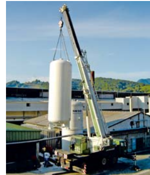
Messer Croatia Plin installed a new oxygen tank at Vetropack.
