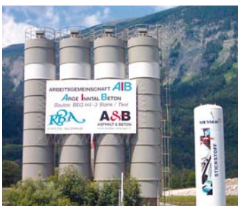
Nitrogen is used for cement cooling.
