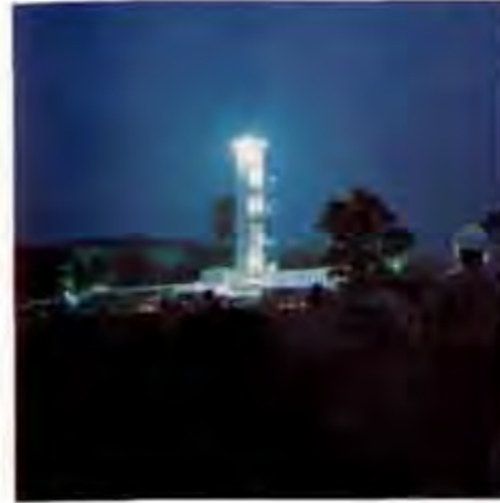
Burdett supplies Western Electric with high-purity nitrogen by pipeline
