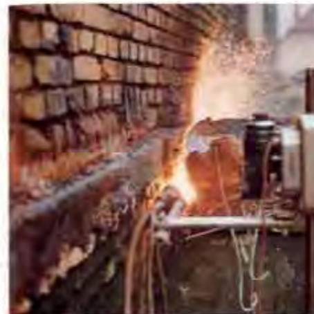
Concrete floor of cinema demolished noiselessly
