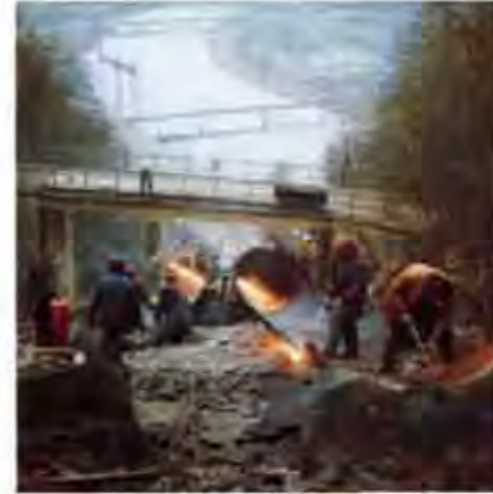
Cast iron water main dismantled with the ESSEN cutting torch
