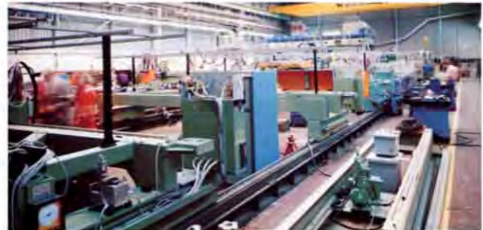
Completion of new assembly shop for flame cutting machines
