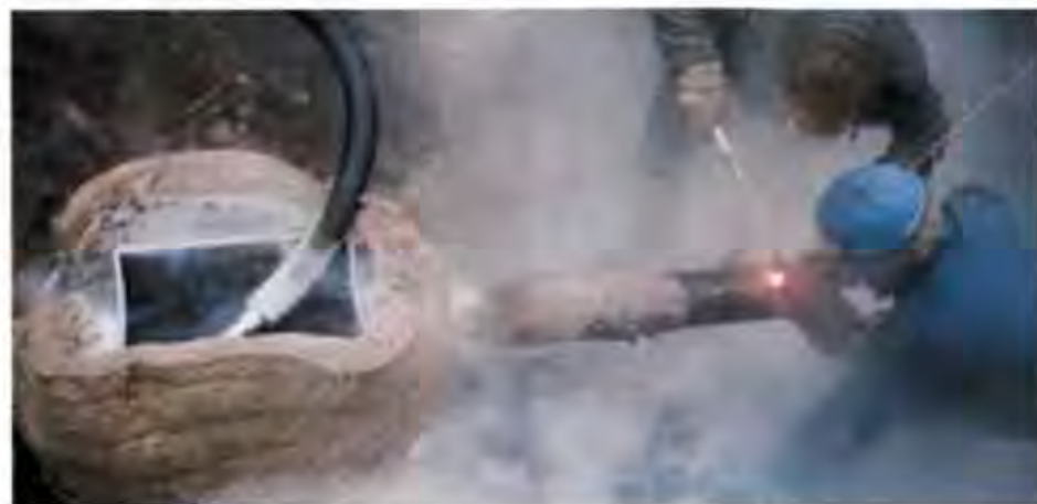
Valve replaced by frozen plug
