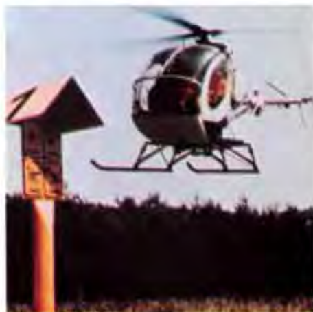
Pipelines for oxygen and nitrogen checked from the air
